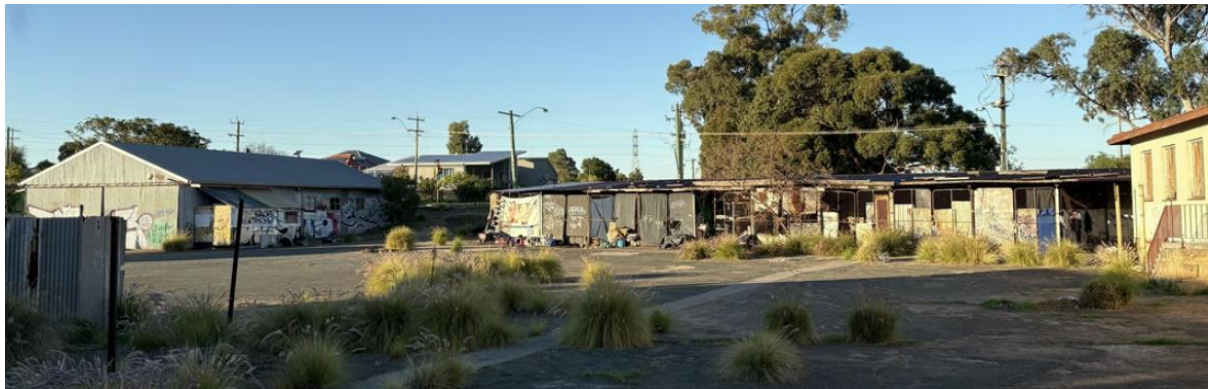
Structures 3 and 4 – to be demolished
