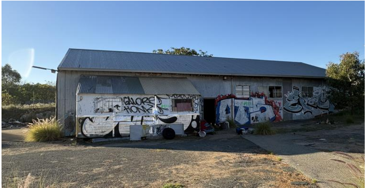
Structure 3 – to be demolished
