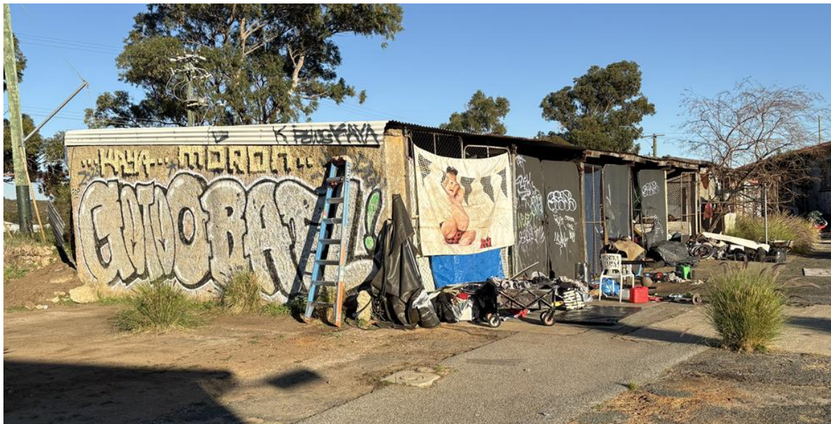
Structure 4 – to be demolished
