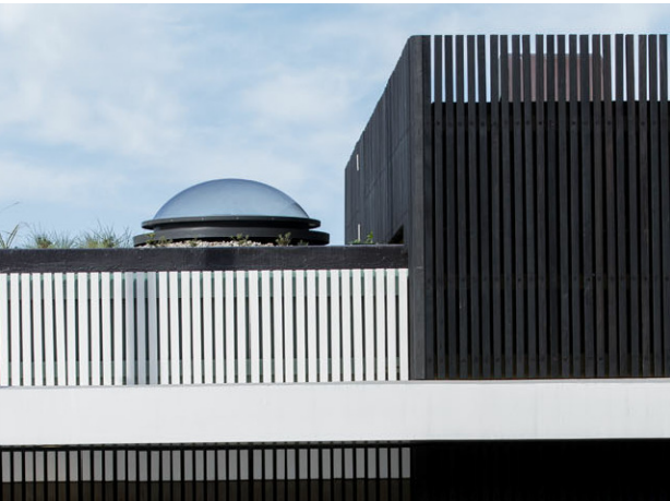
ROOF TOP DOME SKYLIGHTS BRING NATURAL LIGHT INTO CHANGE RMS.
