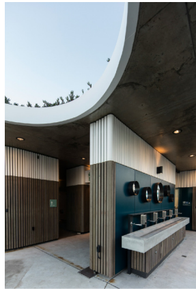
OPEN AIR HAND WASH BASINS
