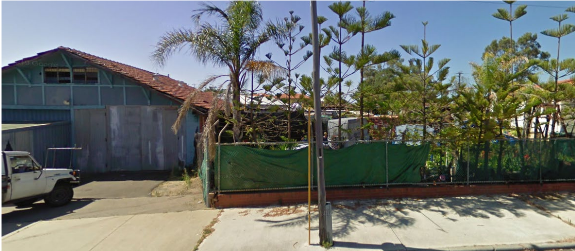
Plate 27. 2009 - South boundary of the Project Area (Courtesy of Google Maps)
