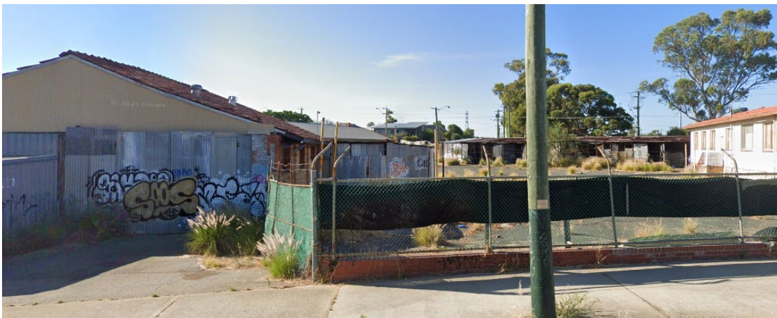
Plate 11. 2025 – South boundary of the Project Area (Courtesy of Google Maps)
