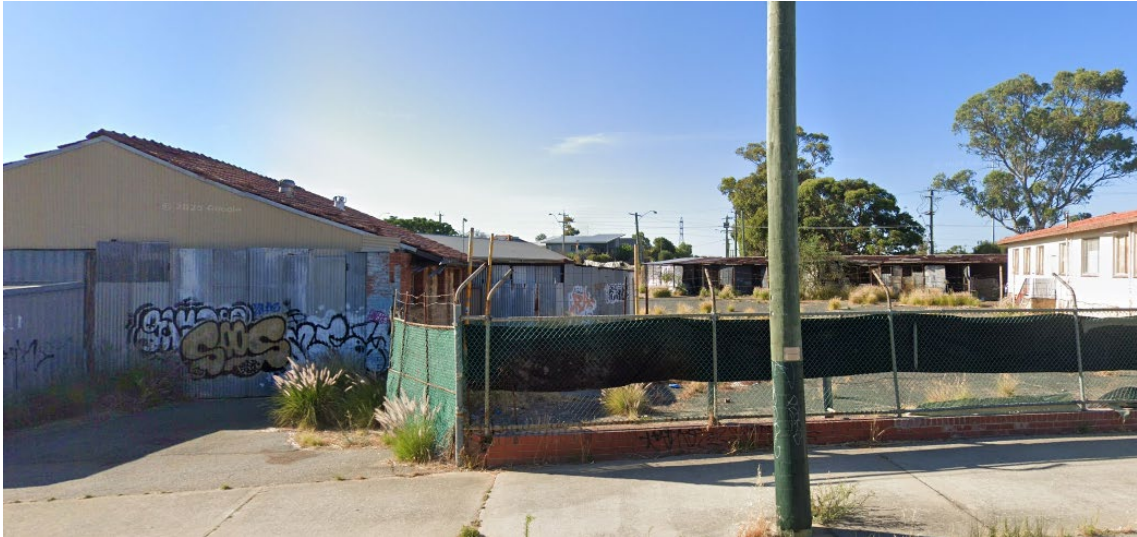
Plate 15. 2021 – South boundary of the Project Area (Courtesy of Google Maps)
