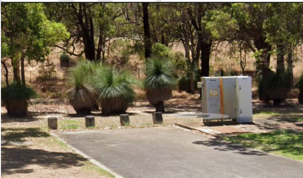
Figure 20: Infrastructure Services located in a Park illustrating an outcome the City seeks to avoid in future planning.
