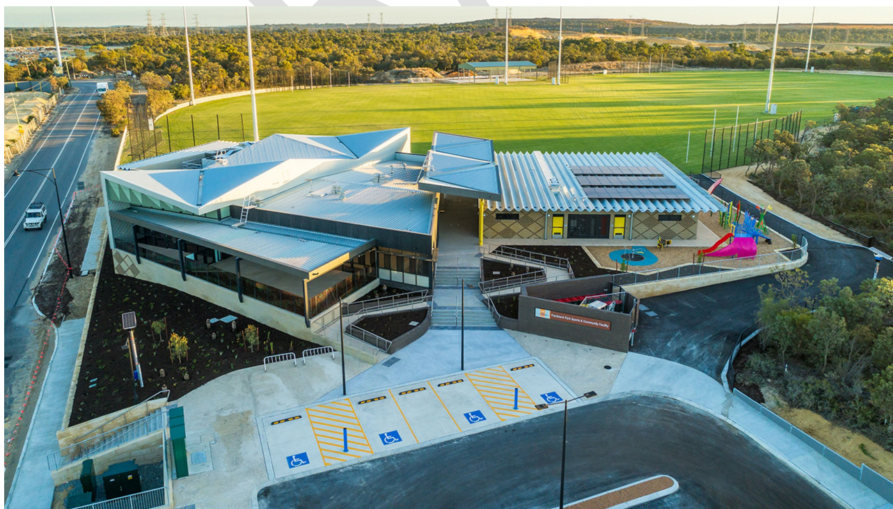
Figure 18: Frankland Park Sports and Community Facility, Hammond Park
