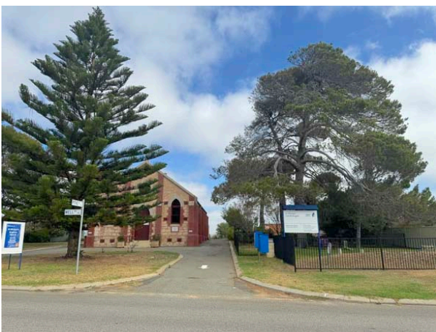
View looking to south showing the centre front pine and west side pines (right).
