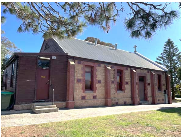
View showing the east side of the Church and the rear lean-to.
