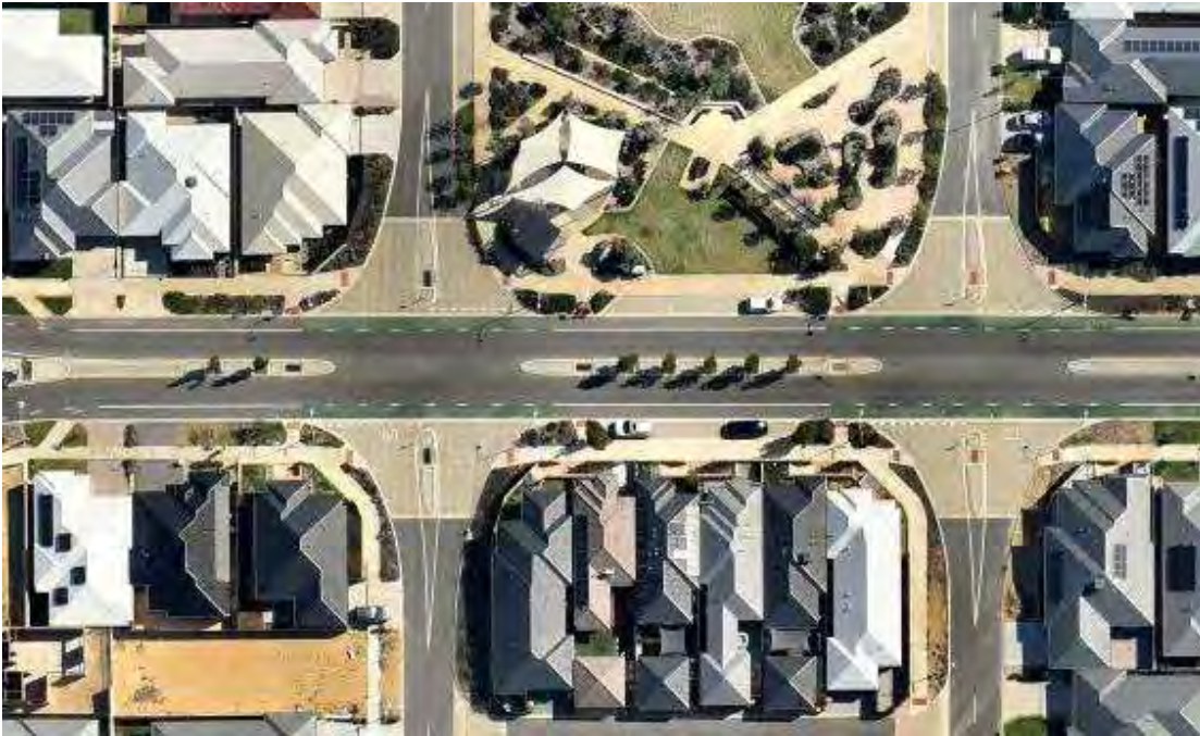
Figure 4-10 A Section of Completed Whadjuk Drive
