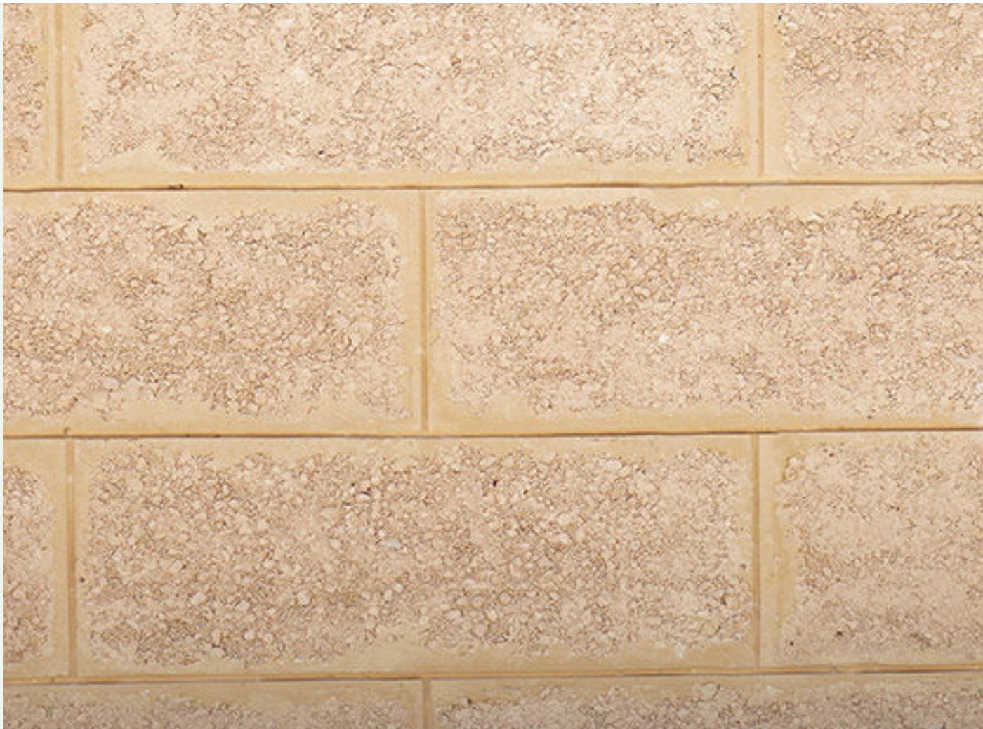
LIMESTONE RETAINING WALLS
