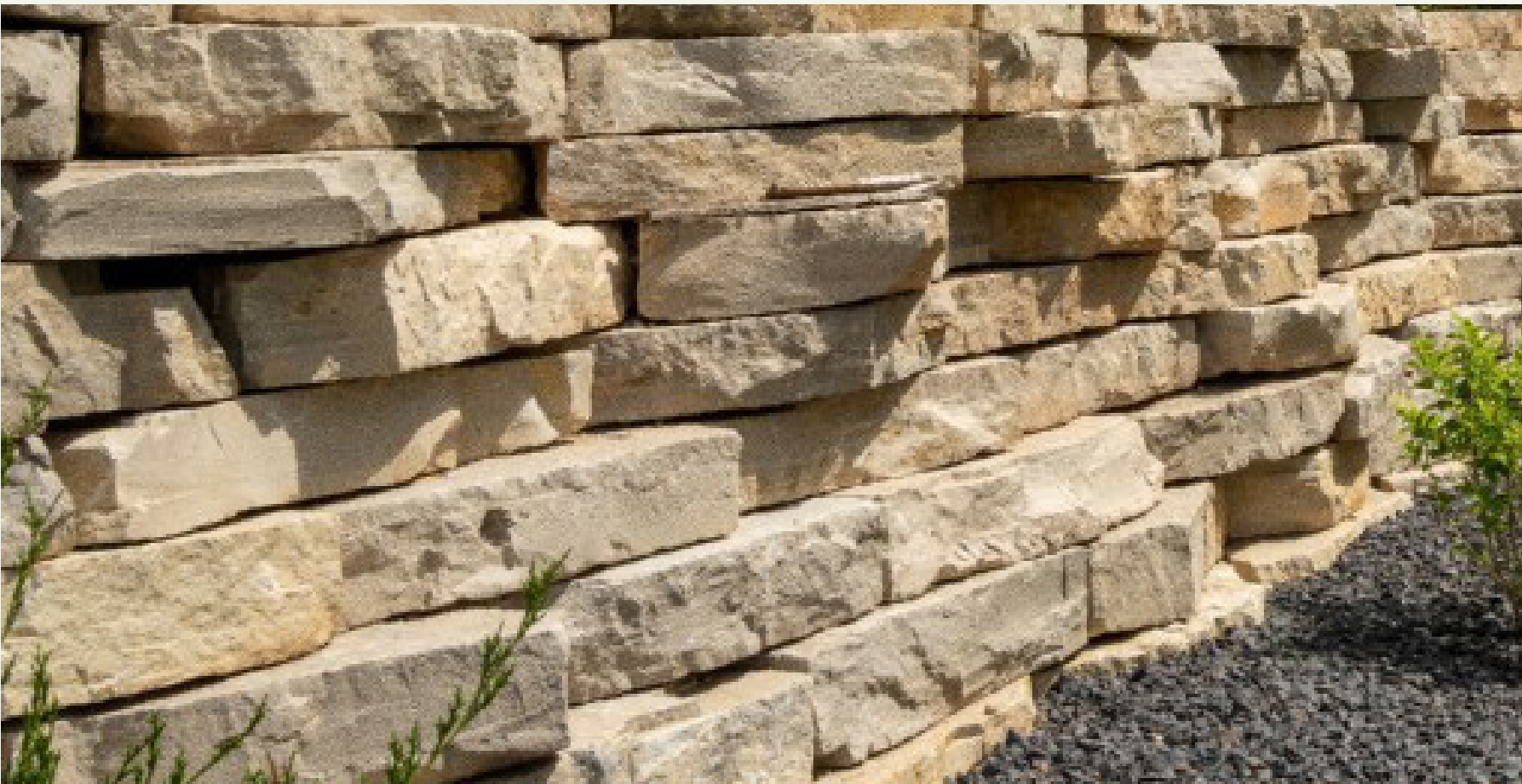
LIMESTONE BOULDERS RETAINING
