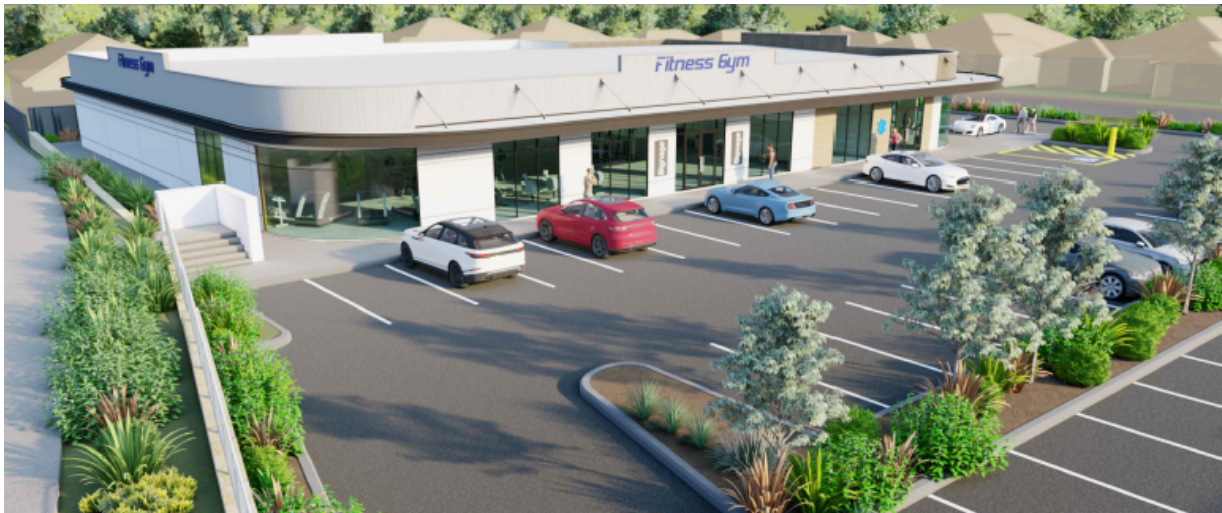
Figure 6 – Western building, as viewed from Russell Road.
