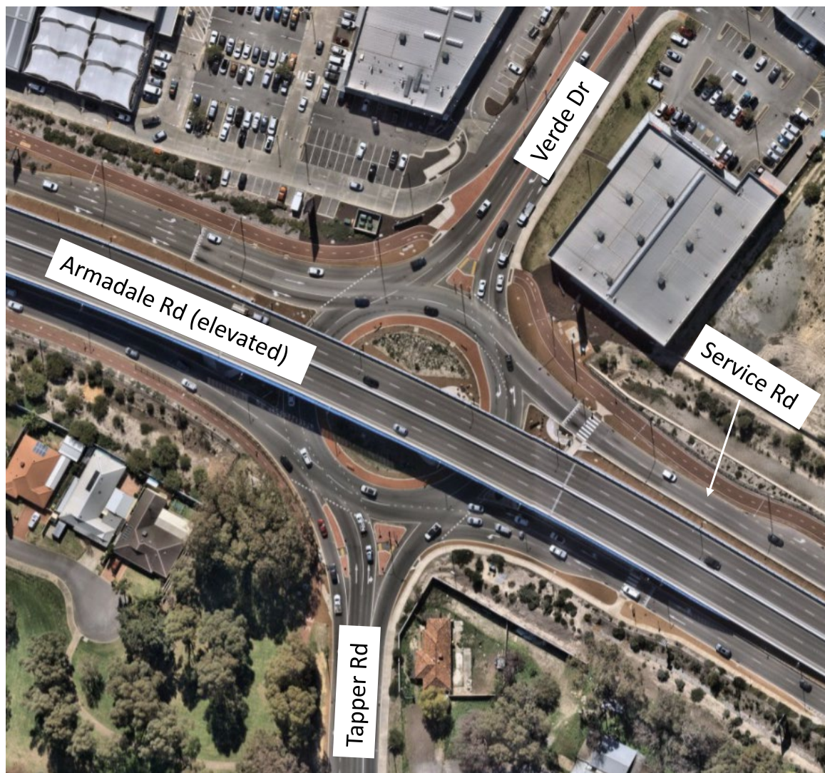
Figure 3: Existing roundabout intersection of Armadale Rd/ Verde Dr/ Tapper Rd
