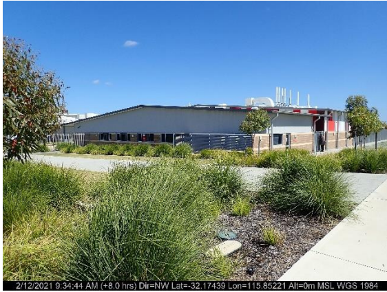
2/12/2021 9:34:44 AM (+8.0 hrs) Dir=NW Lat=-32.17439 Lon=115.85221 Alt=0m MSL WGS 1984 Photo ID: Photo 5 Looking at the low threat vegetation and the school buildings
