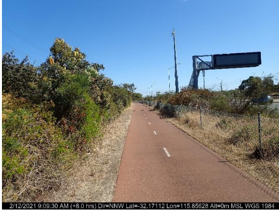
Photo ID: Photo 7 Looking at the scrub, path and freeway.
