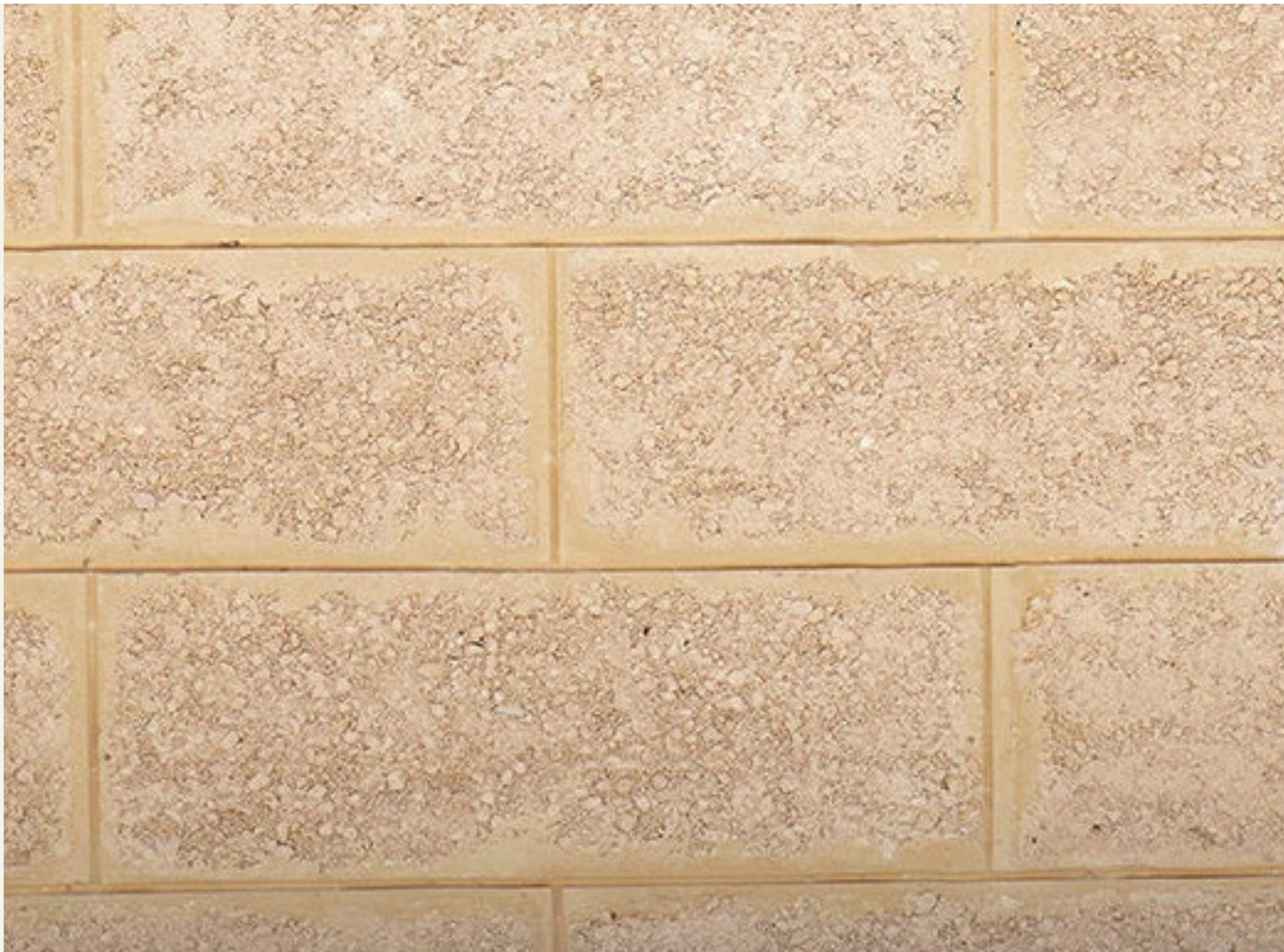
LIMESTONE RETAINING WALLS
