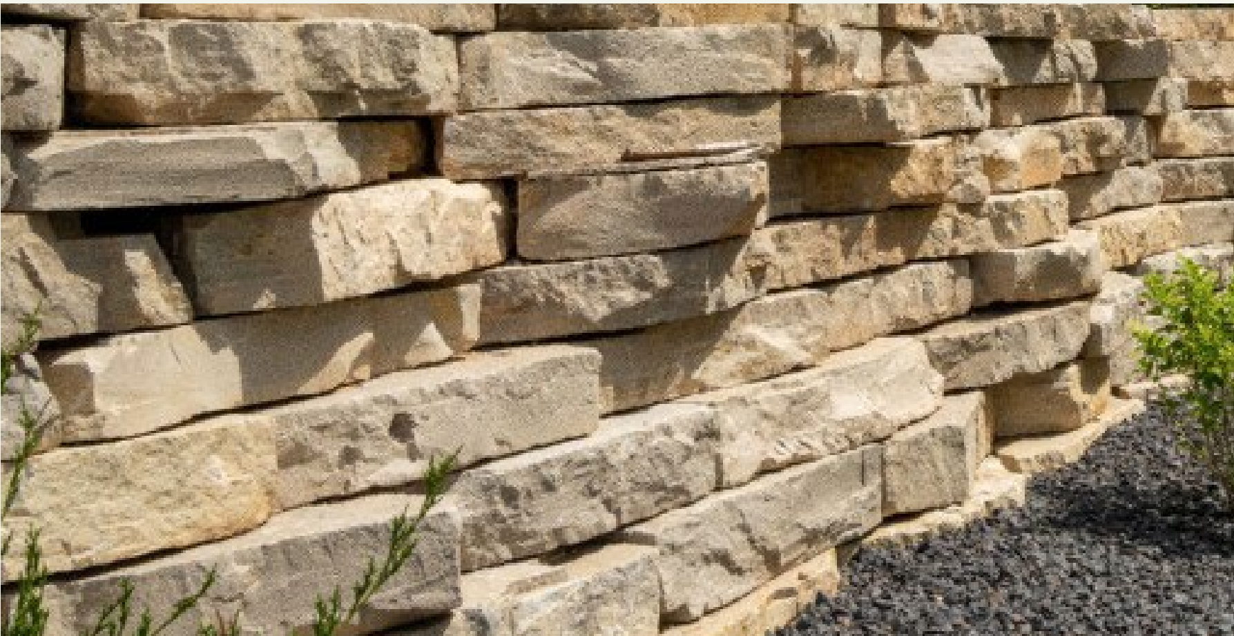
LIMESTONE BOULDERS RETAINING
