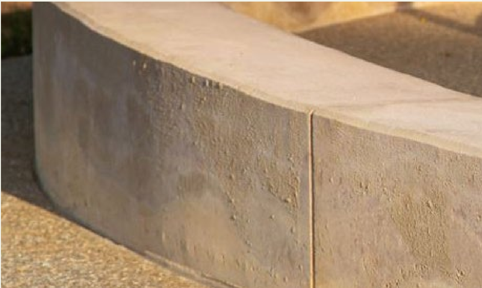
RAMMED EARTH WALL
