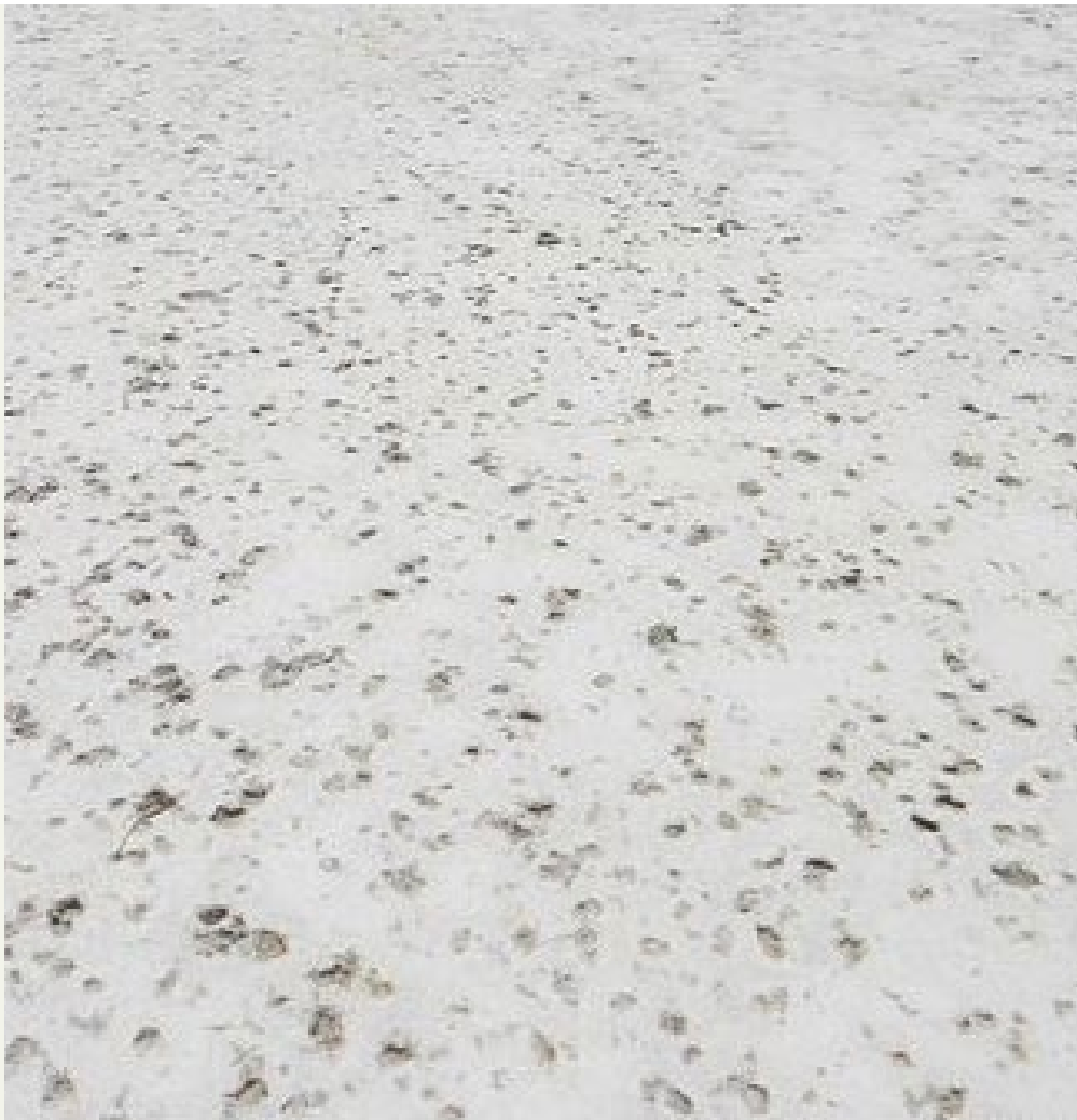
ROCK SALT CONCRETE
